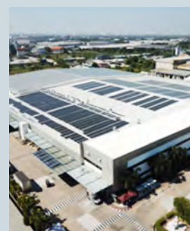
Photo: Solar power generation system (Thai Nippon Seiki)
